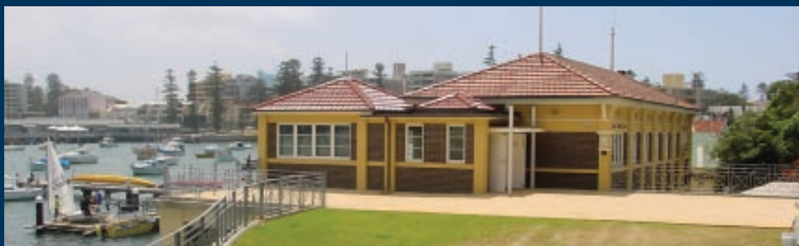
The New Manly Yacht Club Entrance
